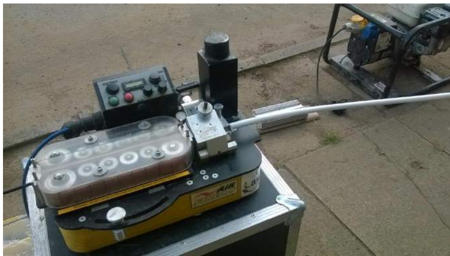
Figure 12: CBS Airstream blowing head (location: EKS substation)
