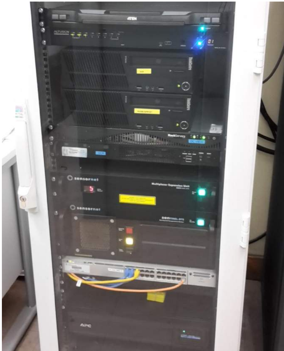
Figure 20: DTS system cabinet at EKS substation
