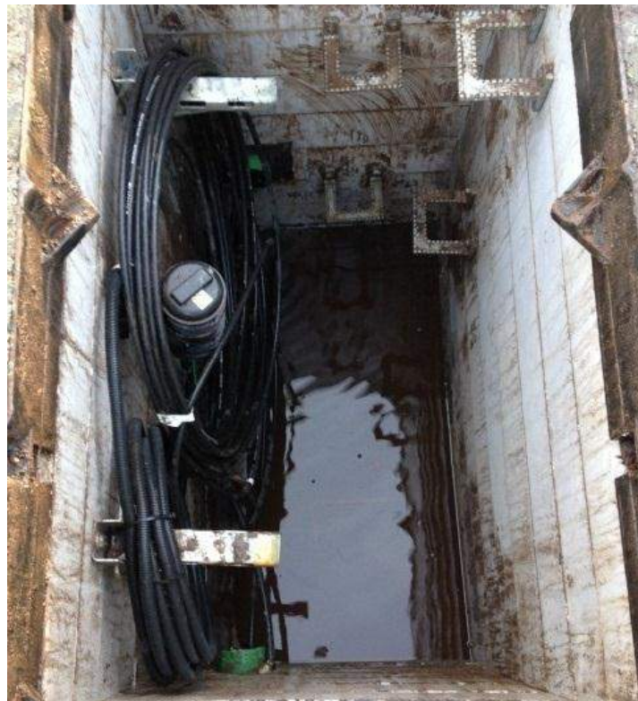
Figure 10: Chamber and DTS fibre joint box
