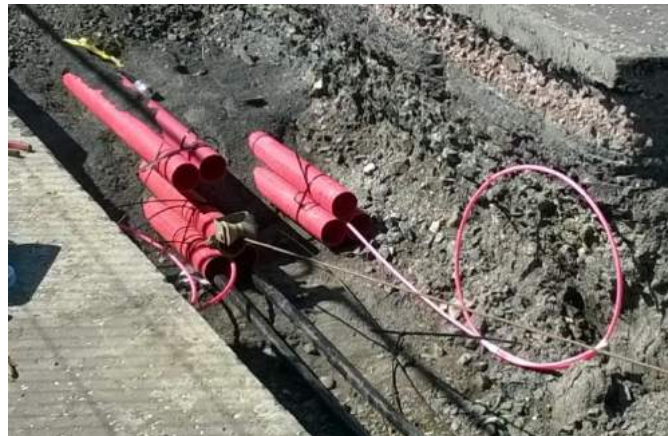
Figure 9: Shared trench with three circuits
