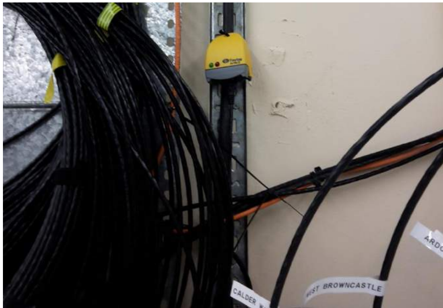
Figure 22: Tinytag located in East Kilbride South substation
