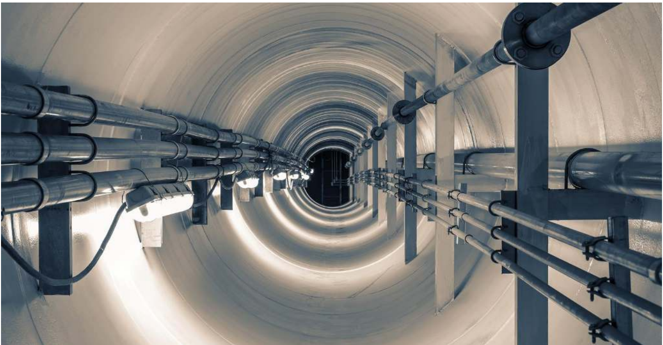
Example of cable utility tunnel containing power and gas lines
