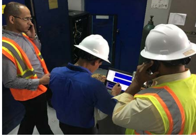
Equipment and personnel in the control room
