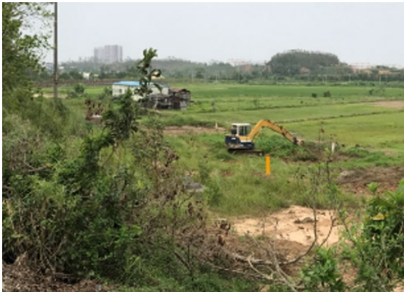
Photo of excavator near pipeline
