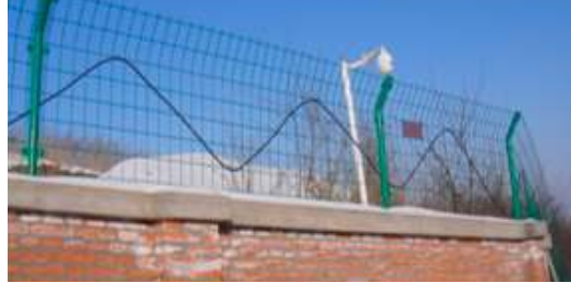
Example of fence section with sensing cable installed >>
