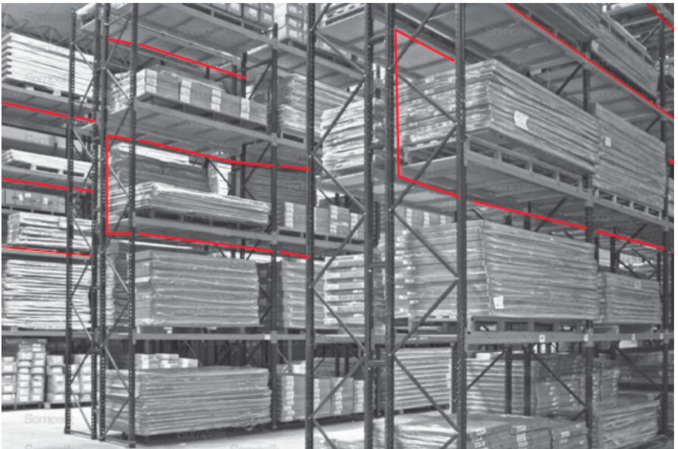
Figure 1 Installation of LHD cable on the racks
