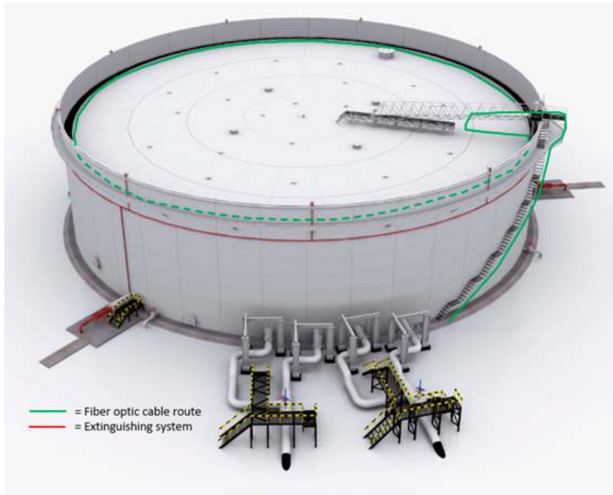
Figure 3: Cable route around tank
