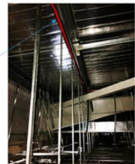
Fiber optic linear heat detection cable in ceiling void
