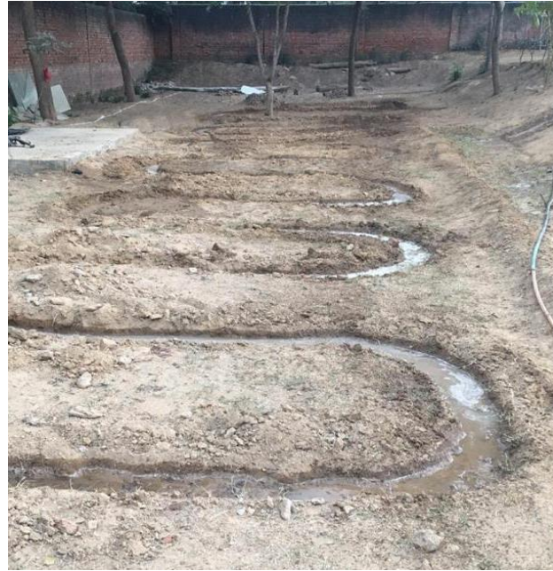
Figure 7 - Covert buried detection – patterns
