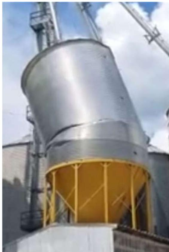
*Figure 1 - Example of failed coil silo*
