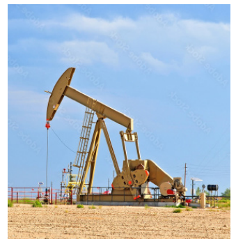
Well heads, block valves and pumping stations
