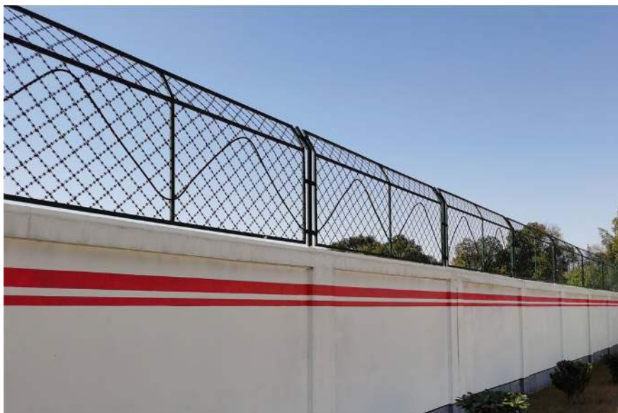
Figure 4 - Photo of cable mounted on fence topper section in serpentine formation
