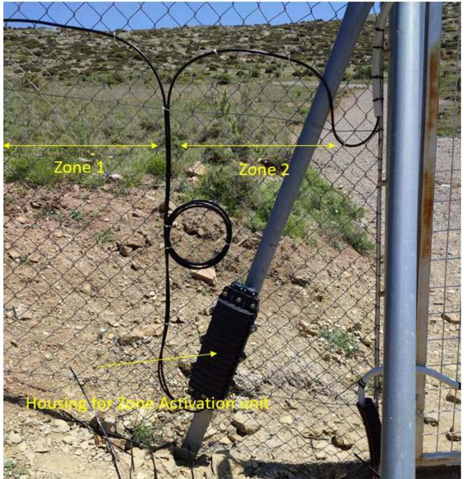
As this was a very remote site, there is no on-site control room but a small equipment enclosure which is not climate controlled. The ZoneSentry units are rated to 70°C and so can survive in even the harshest conditions. The image (right) shows details of the remote equipment enclosure on site.
