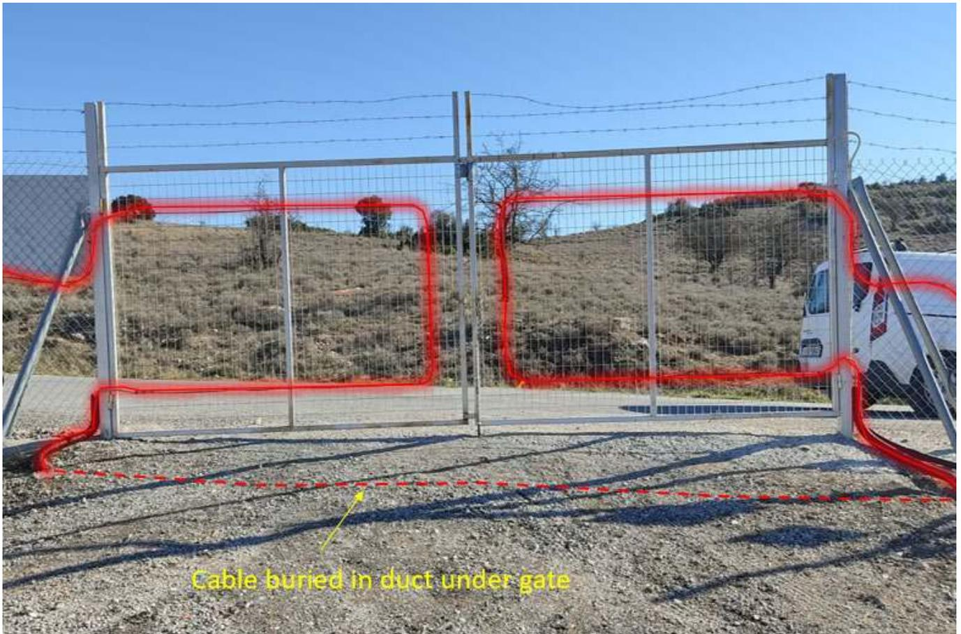
*Figure 3 - Example of sensing cable installation on gate*
