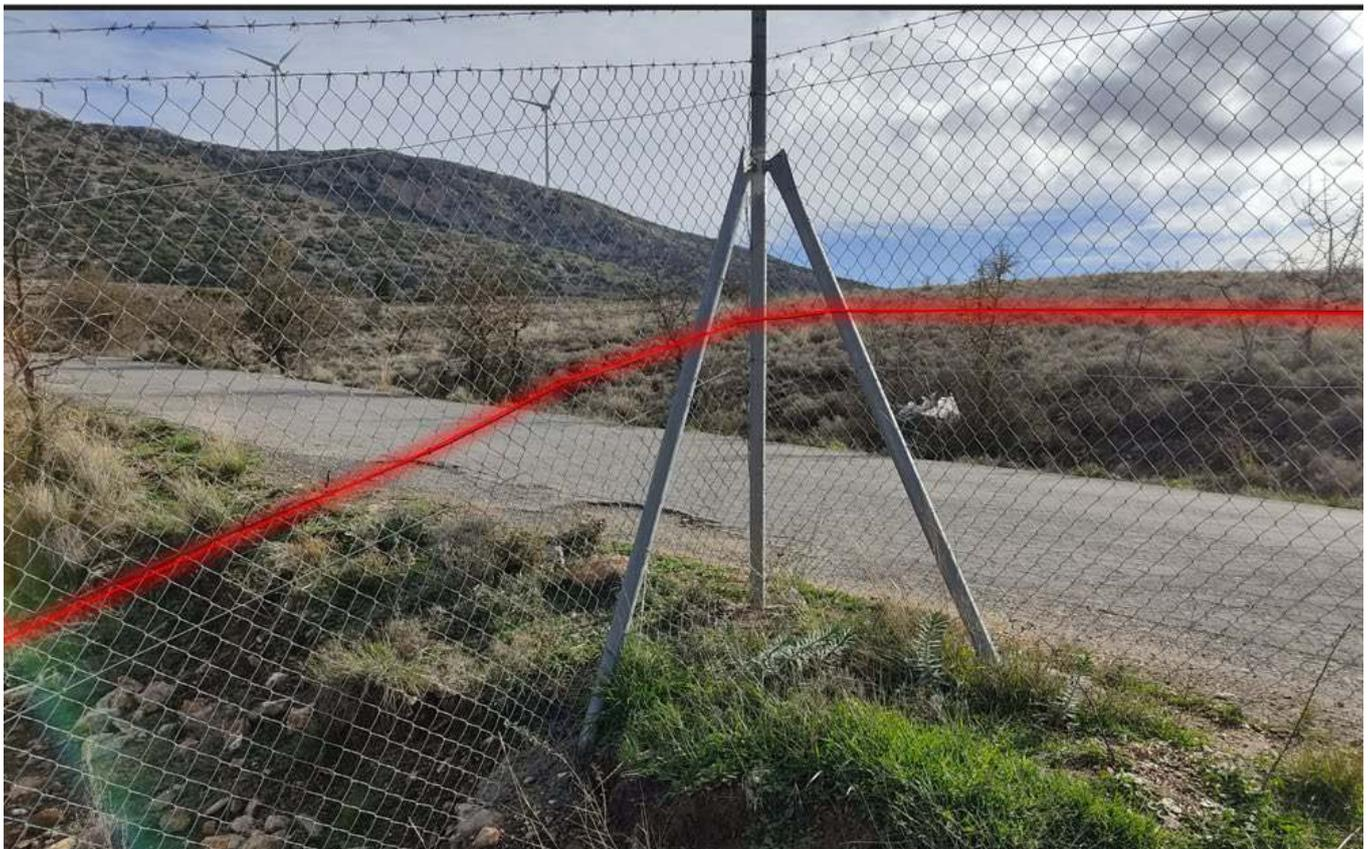
*Figure 2 - Fiber optic sensing cable position on Fence*
