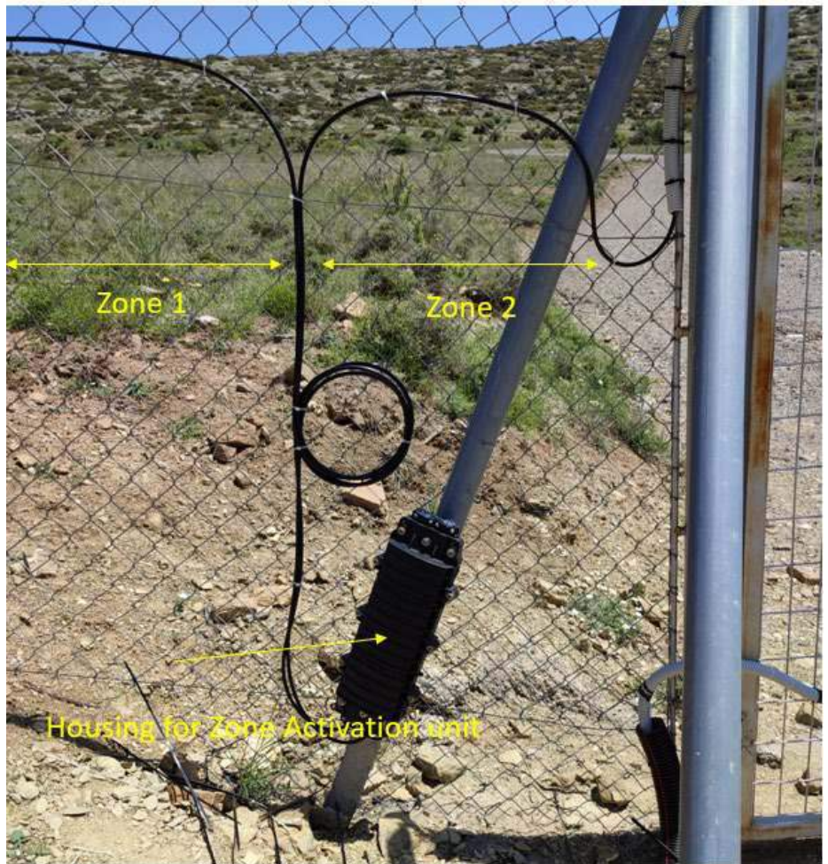
Figure 4 In field splice housing
