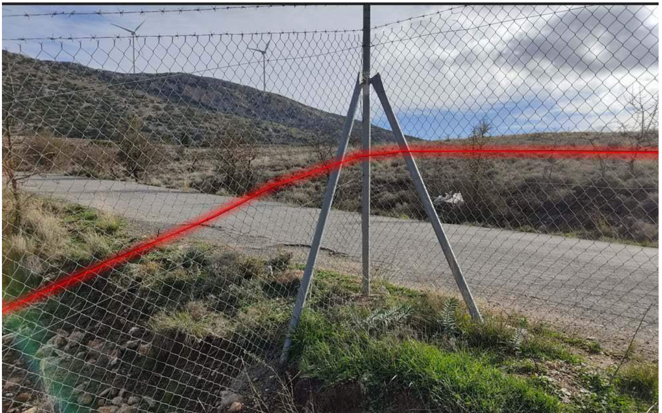
Figure 2 - Fiber optic sensing cable position on Fence
