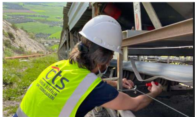
Installation of the sensing cable
