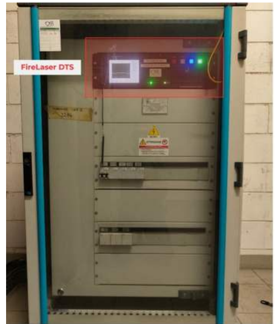
Figure 2 - FireLaser Installation
