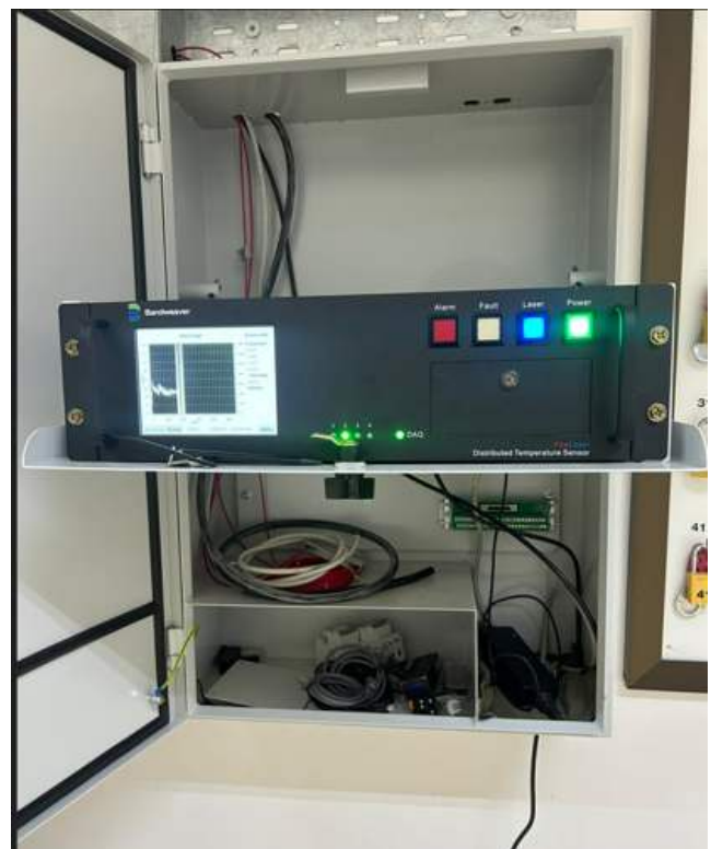
Figure 3 - FireLaser installed in wall mounted cabinet
