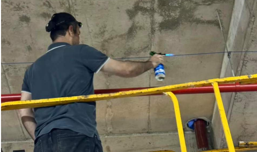
Figure 7 - System testing on site
