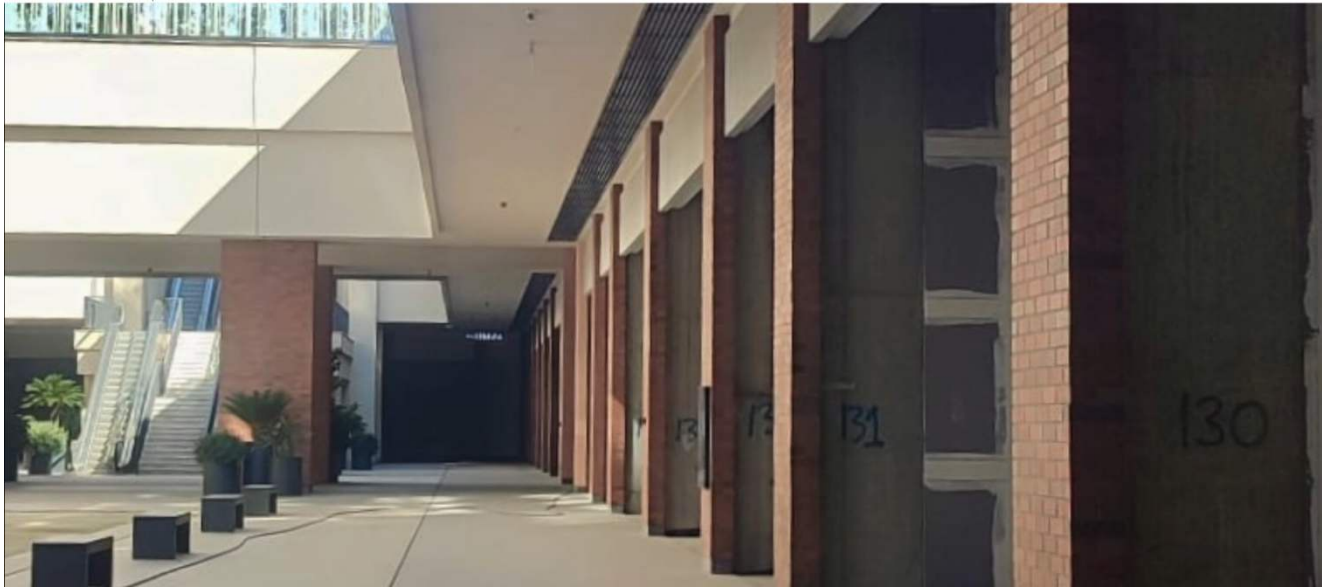
Figure 2 - Photo of suspended ceiling run
